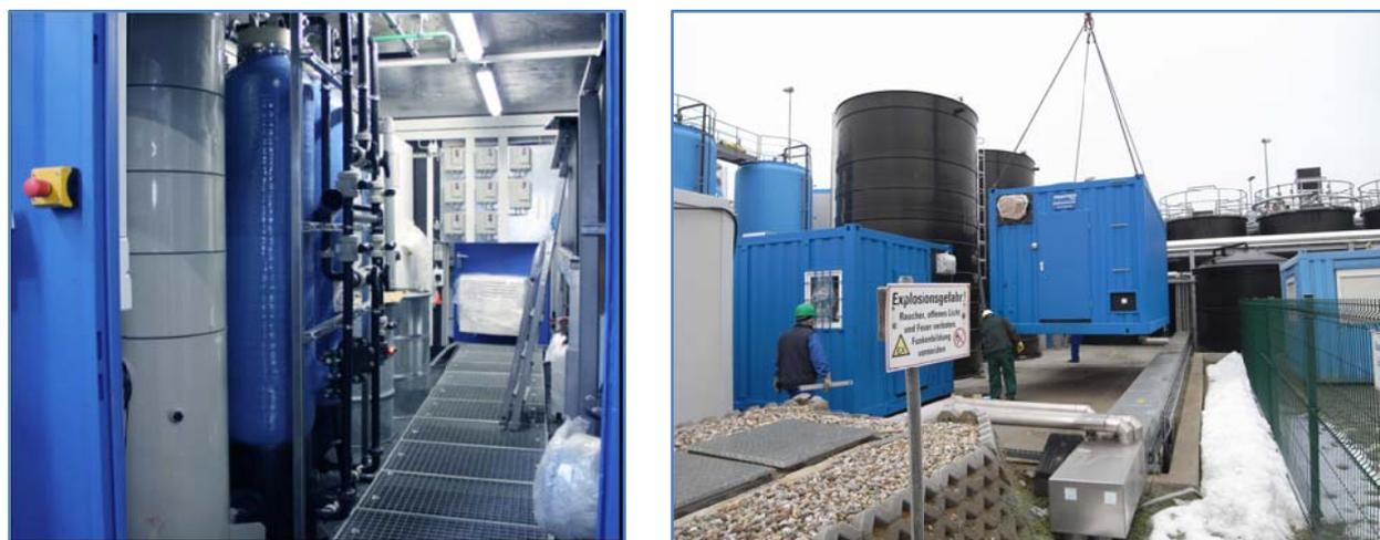
**Fig. 1:** View into one of two *Treatment Train* containers and placement of the units at a field site for plot testing.
